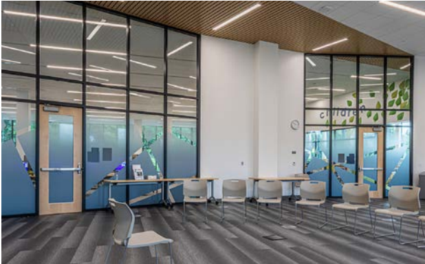
Meeting Room with graphic window film to provide light and movement with some privacy
