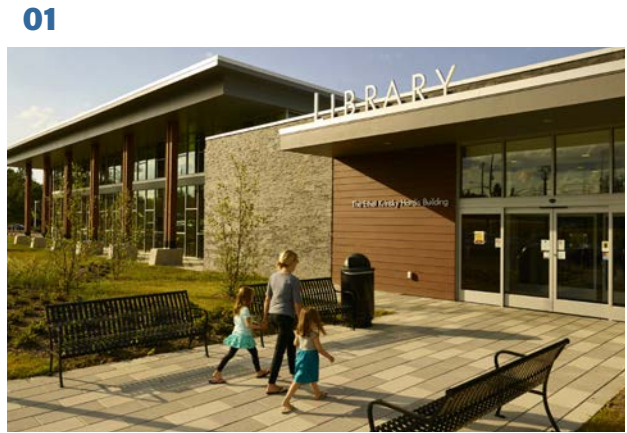
Entry plaza / walkway with benches and automatic bi-parting doors
