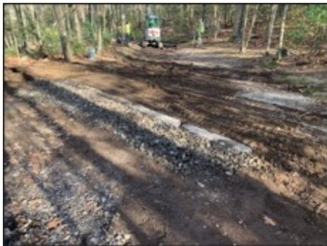
Improvements to the Case Mountain trail and path to the summit were made. The Department repaired washouts and installed water breaks to prevent future washouts and reduce their severity.
