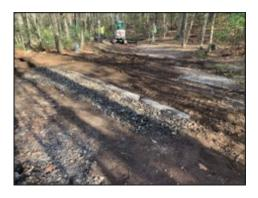
Improvements to the Case Mountain trail and path to the summit were made. The Department repaired washouts and installed water breaks to prevent future washouts and reduce their severity.
