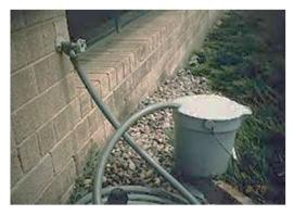
A common Cross Connection found at home is a garden hose submerged in a bucket containing a non-potable substance.
