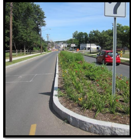
Figure 7: The Broad Street reconstruction work provided significant infrastructure upgrades to the area. Work included creating a uniform street width along the entire roadway, constructing uniform curbing and sidewalks on both sides of the street, eliminating unnecessary curb cuts to improve traffic flow, improving storm water management, milling and repaving the entire street and various landscape improvements.
