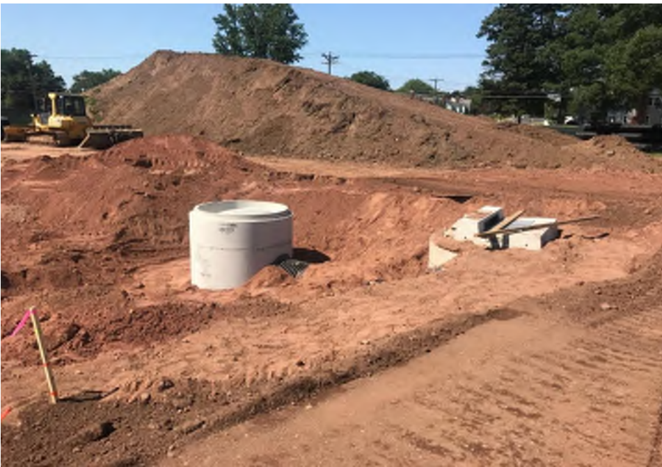
More site drainage and sewer by Richard (stiework)
