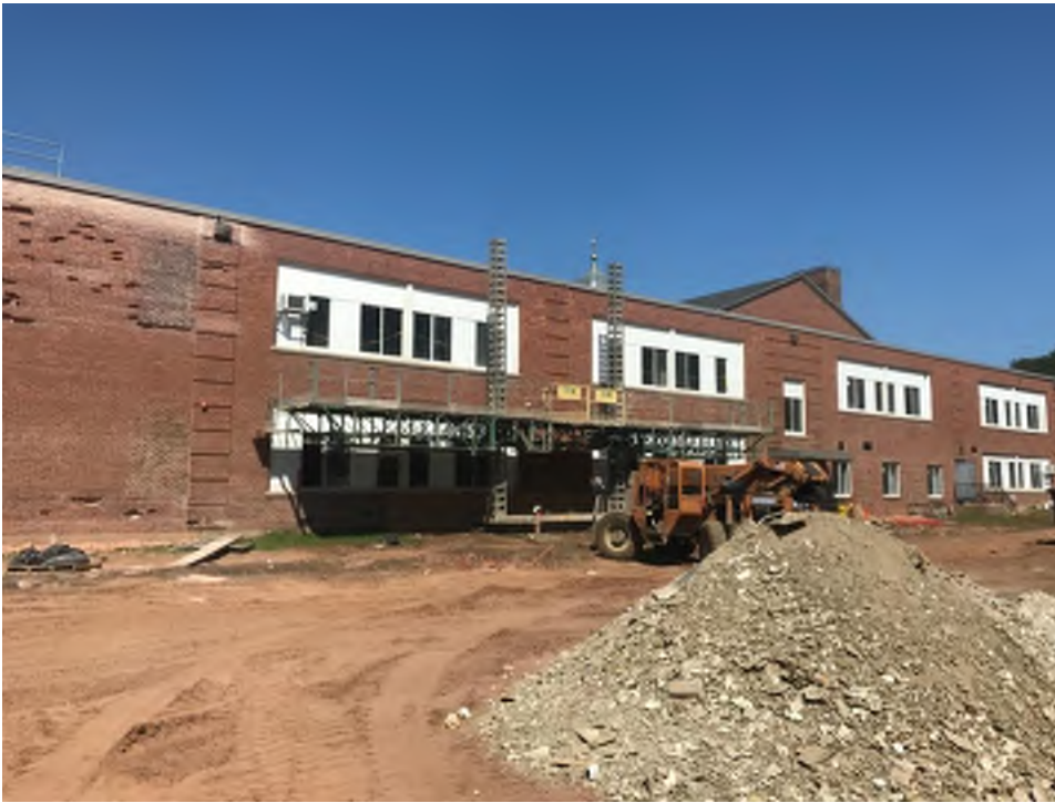
CT Mason (masonry) has started the brick cleaning and masonry reappointing.
