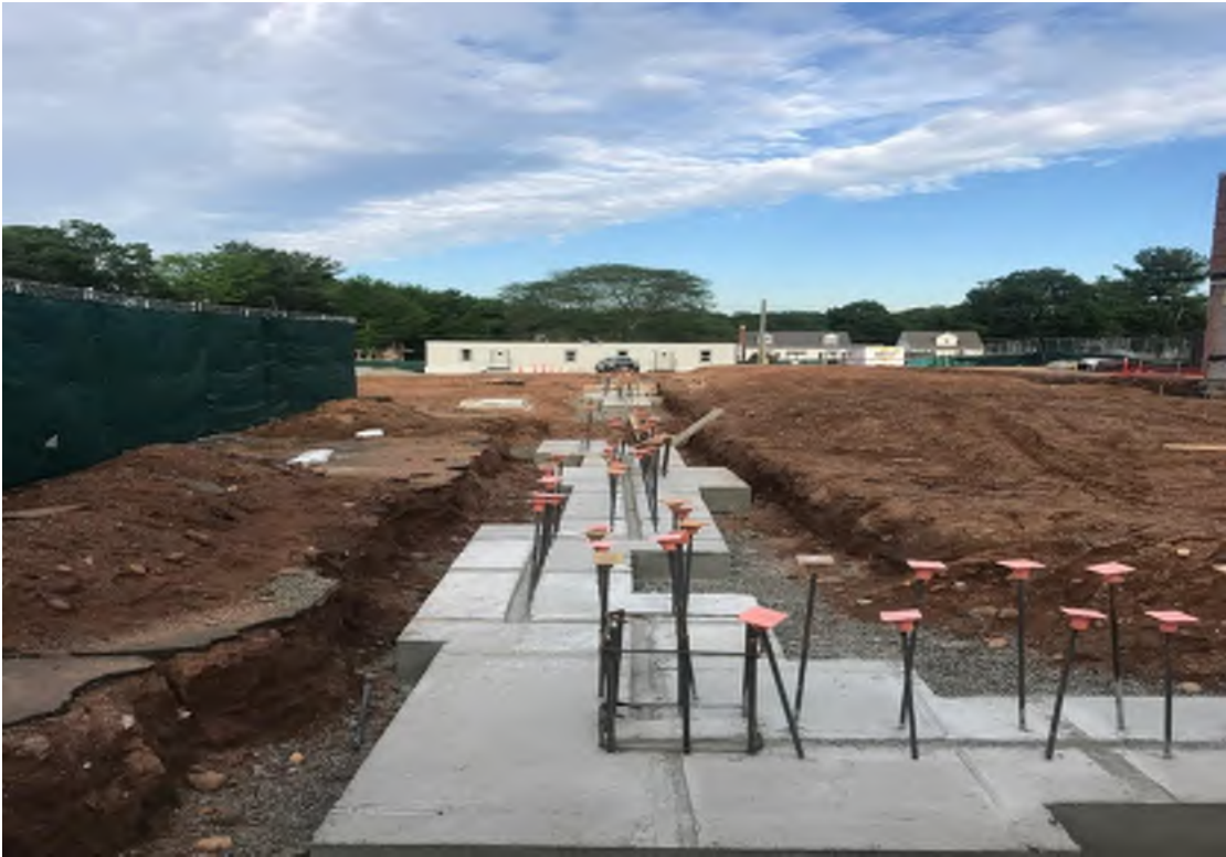
Footings that have been placed and poured.
