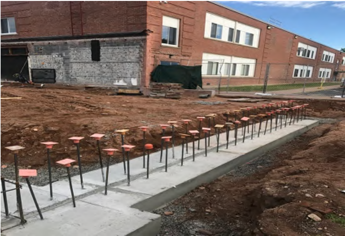
Footings that have been placed and poured.
