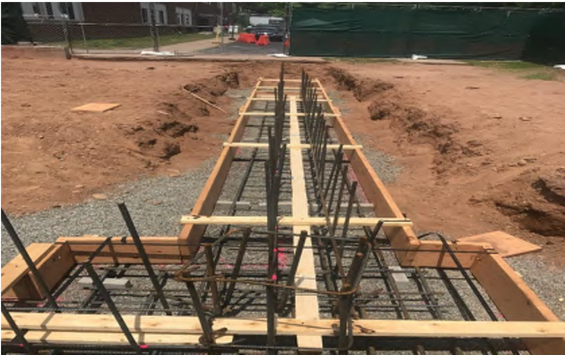
Footings been formed with rebar placement
