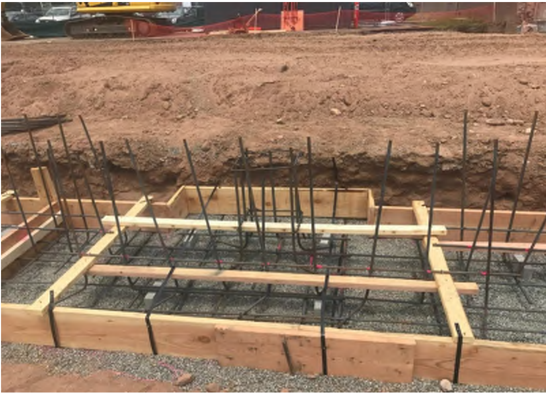
Rebar installation at footings.
