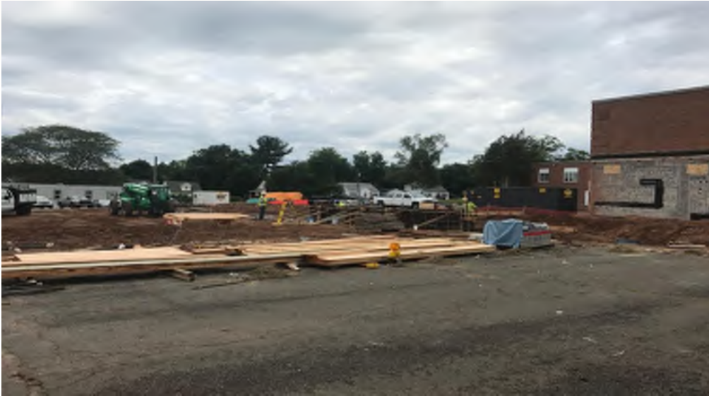
MT Ford (concrete) prepping and forming foundation walls.
