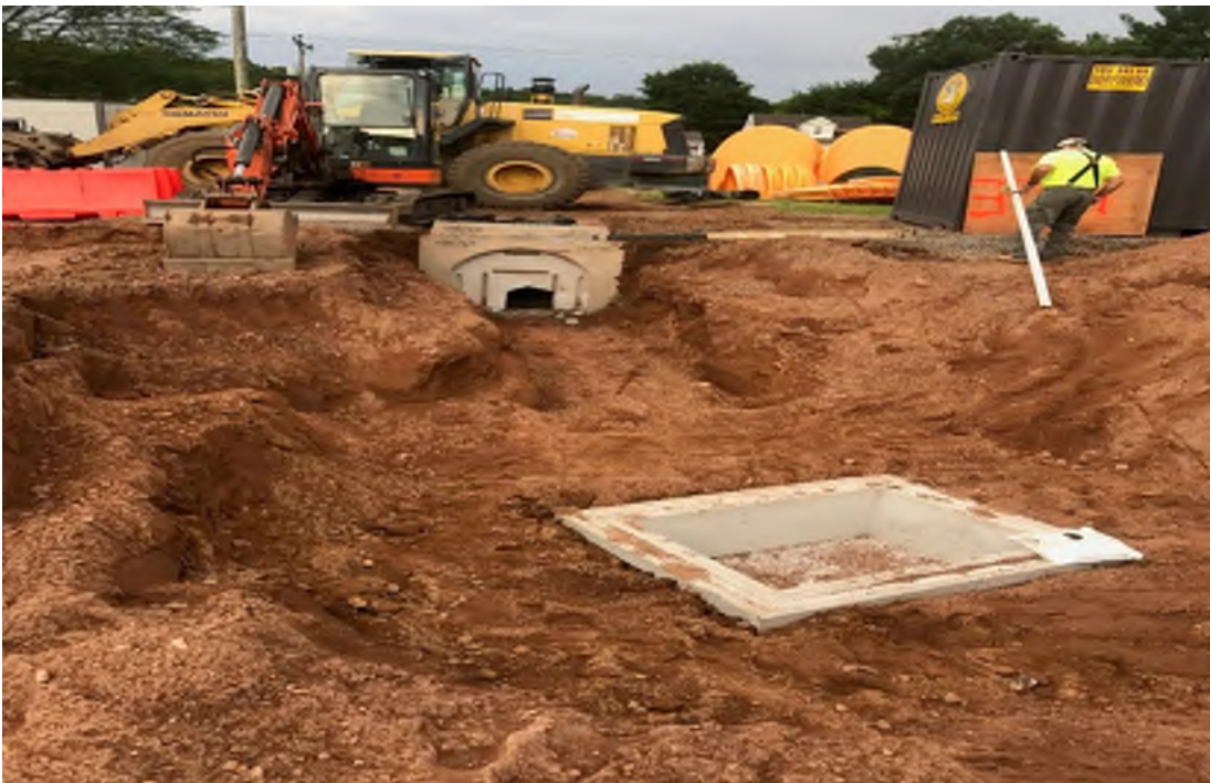
Richards Corp (sitework) installing new storm drainage.
