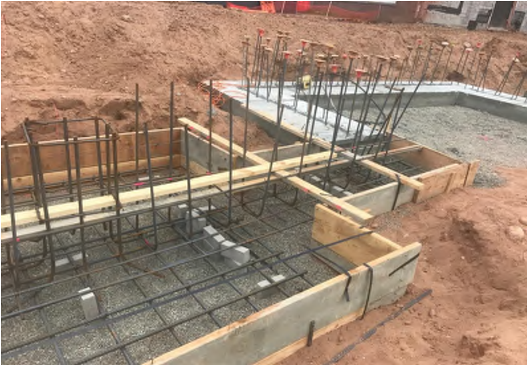
Rebar installation continues at footings progression.
