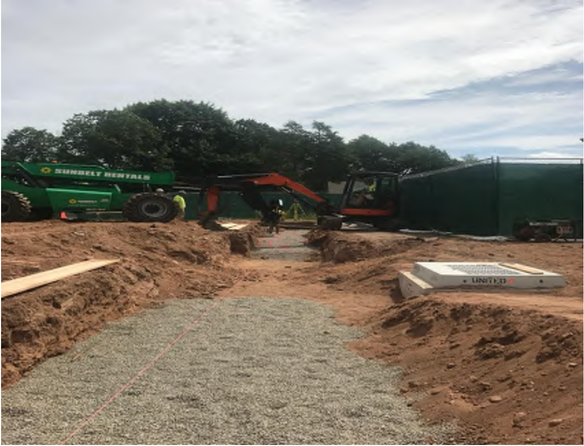
Excavations for foundation footings.
