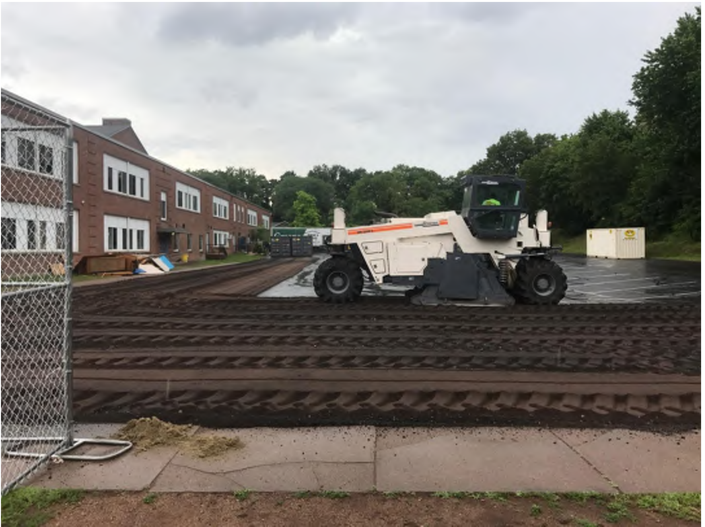
Back parking lot being reclaimed. Areas have been left paved until building move out is completed.
