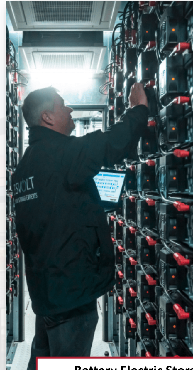
Battery Electric Storage (BES) Emergency power and demand reduction
