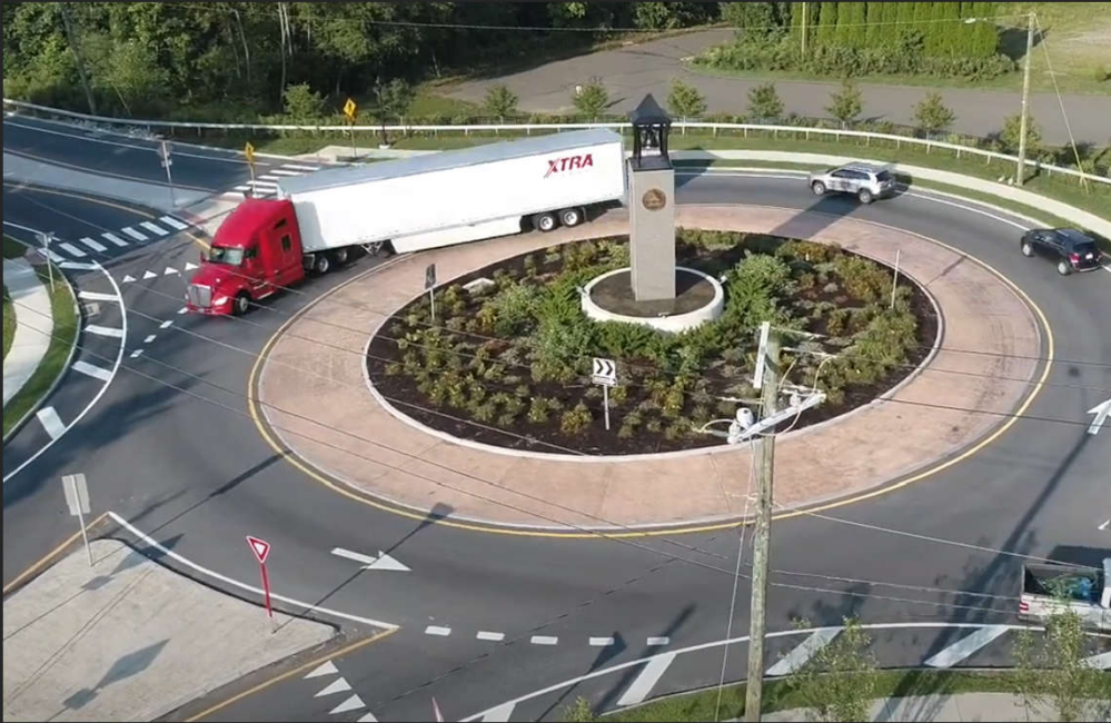
Designed to accommodate tractor trailers and emergency vehicles
