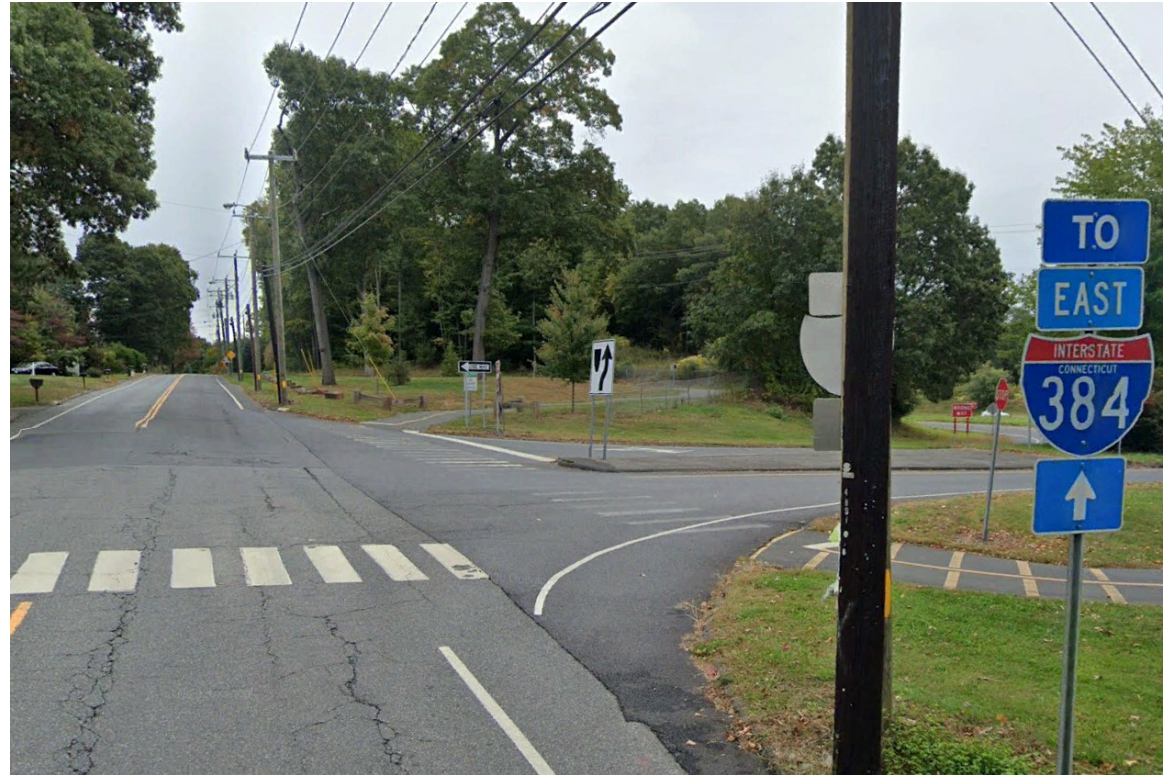
Figure 3.28: Faded crosswalk markings at I-384 ramp crossing of the Charter Oak Greenway. Pavement markings on the pathway, installed at the same time, remain in good condition. Image credit: Google Earth
