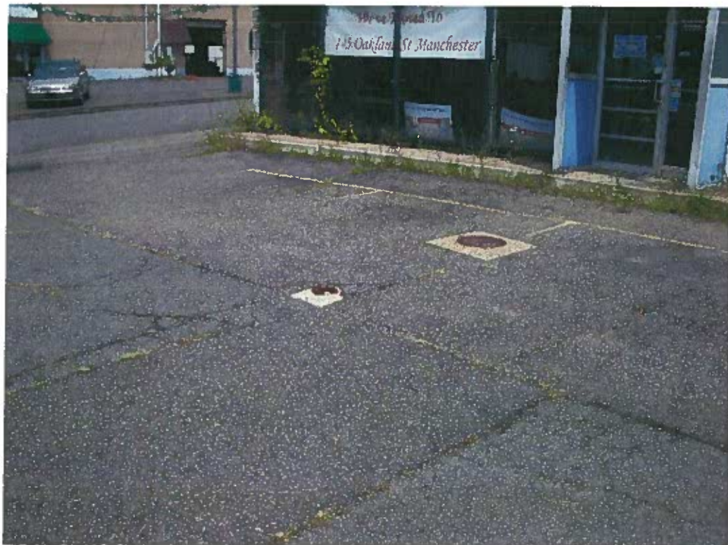
Location of a UST located adjacent to west of the Site building
