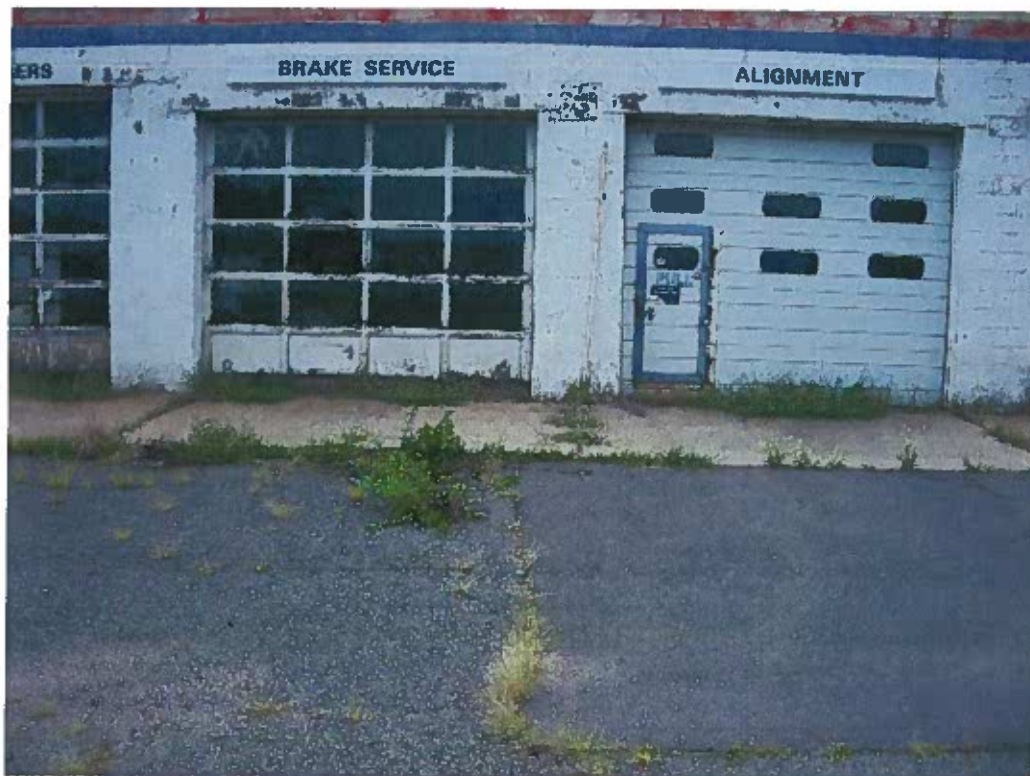
Location of a UST located adjacent to the south of the overhead doors
