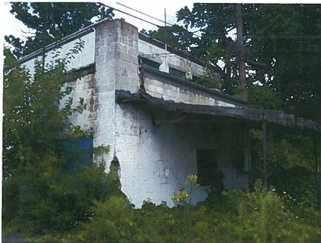
Former storage area located adjacent to the south of the boiler room
