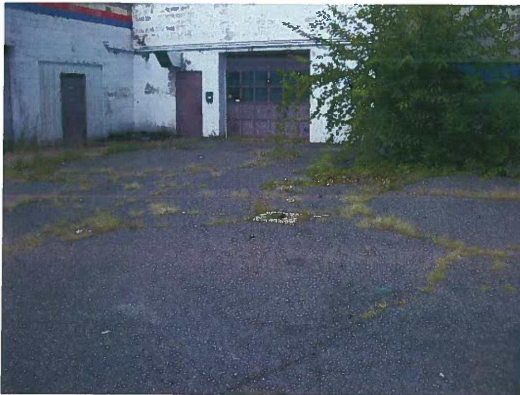
Location of the 6,000-gallon heating oil UST located adjacent to the west of the boiler room
