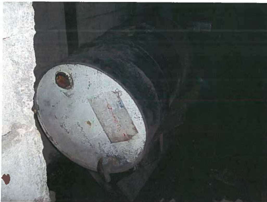
Empty 55-gallon drum located against the eastern wall of the boiler room
