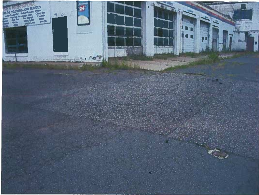
Location of two USTs located adjacent to the southwest of the Site building
