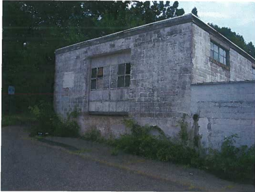
A loading dock located in the northwestern portion of the building
