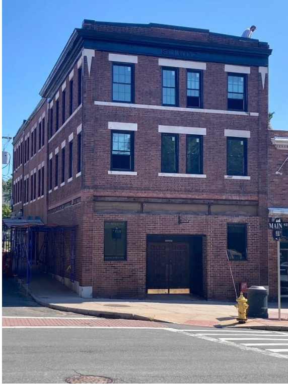
2-4 Pearl AKA 623 Main Rehabilitation
