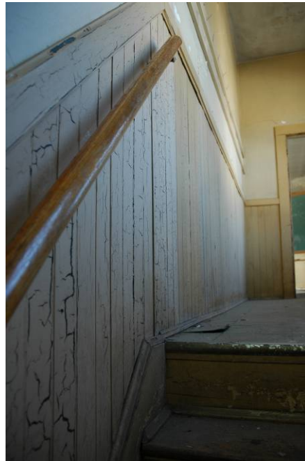
View of Stair
