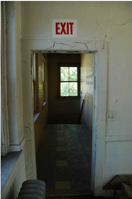
View of Stair
