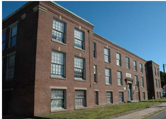
Cheney Building – Front Elevation
